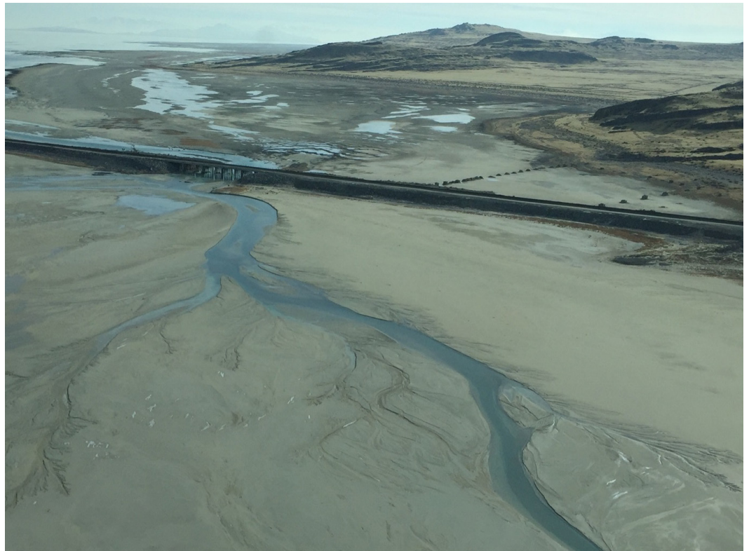
Aerial photo of the railroad causeway that bisects the Great Salt Lake.
